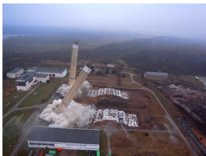
Demolition by blasting of two smokestacks near "Luther town" Germany
