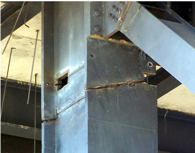
*Fig. 5: improper cut*
