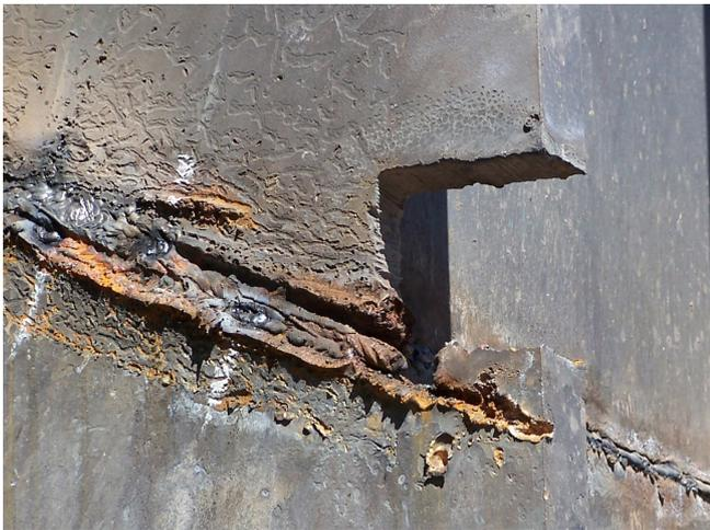
*Fig. 7: insufficient cut after blast (attempt)*
