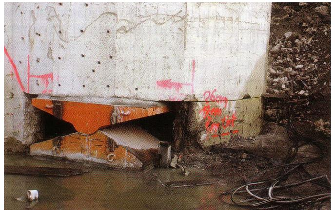
*Fig. 9: steel hinge*
