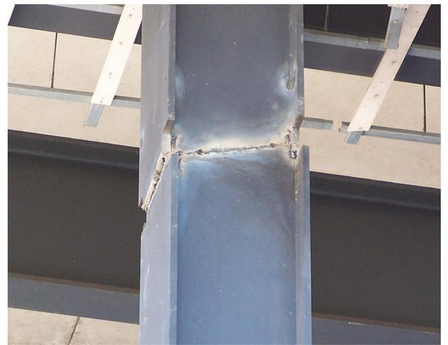
*Fig. 6: improper cut*
